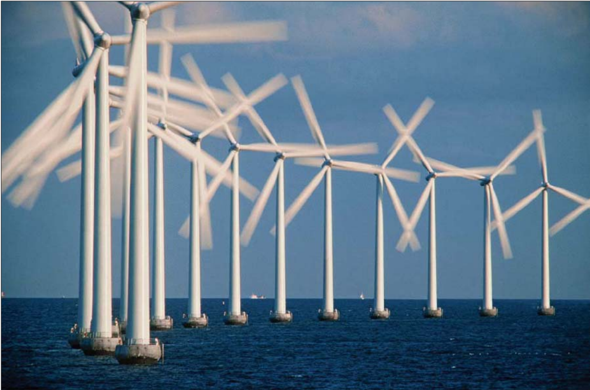
Fig. 3. Submarine cable HVDC routes are of great interest in view of the large offshore wind parks that are planned.
